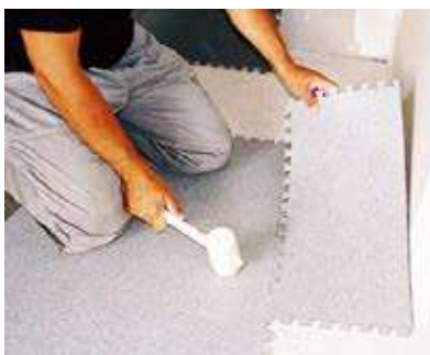
Clic System Planks, Attraction, GTI... → unique looselay tiles and planks with no adhesive.
